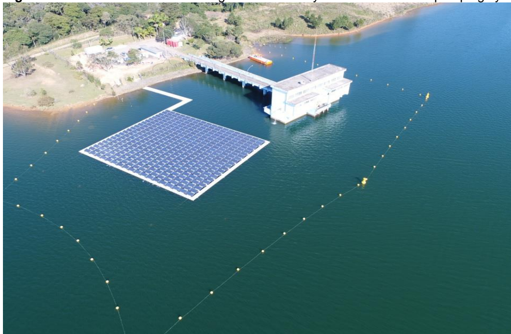
Figure 12 – Aerial view of the Floating Photovoltaic System and the water pumping system
