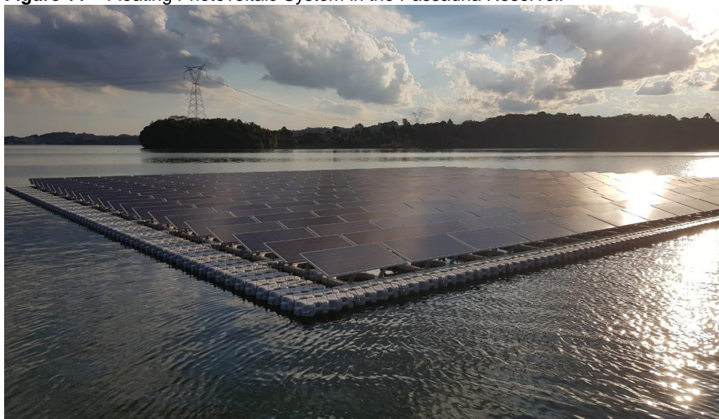
Figure 11 – Floating Photovoltaic System in the Passaúna Reservoir
