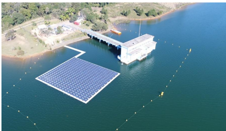
Figure 21 – Aerial view of the Floating Photovoltaic System and the water pumping system
