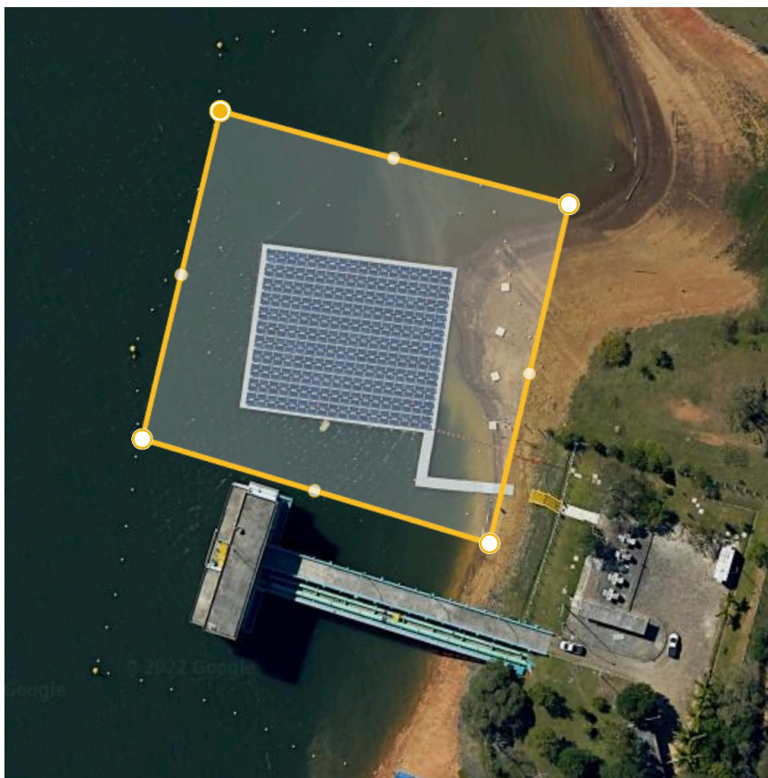
Figure 5 – Aerial view of the Floating Photovoltaic System in the Passaúna Reservoir and the area of interest
