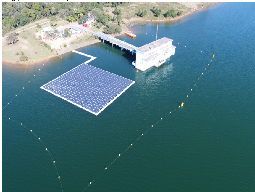
Figure 8 – Floating photovoltaic system at Passaúna reservoir
